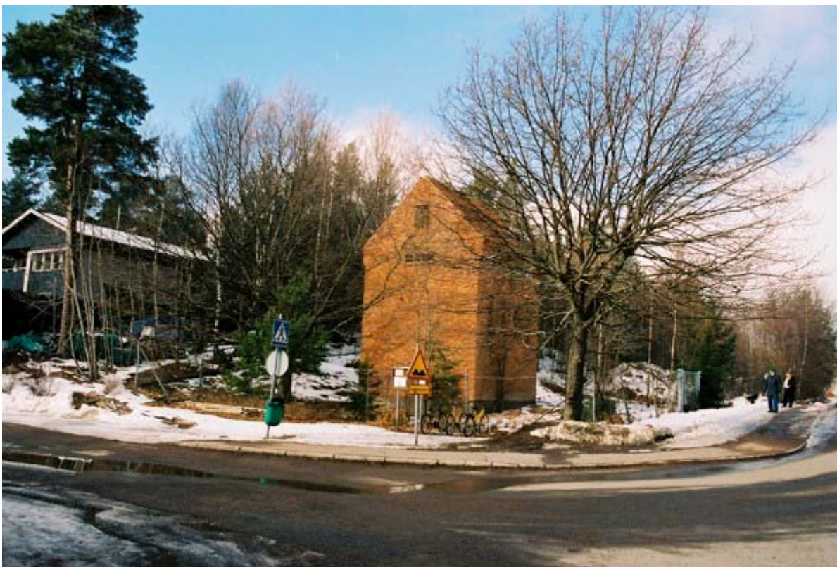
8 Rindö 3:265, Transformatorstation, fr Ö.
